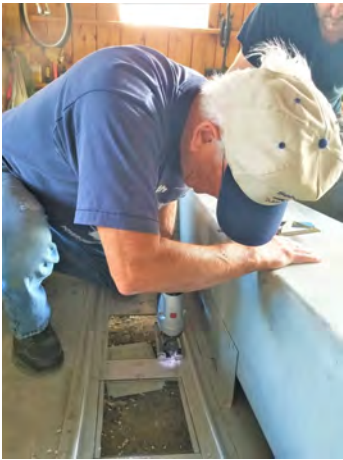
Brian Woodworth cutting the openings for the viewing windows
